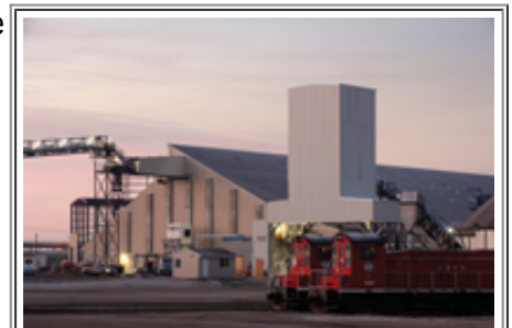
Locomotives stand ready to load unit trains at the new Lange-Stegmann St. Louis Urea Center.
